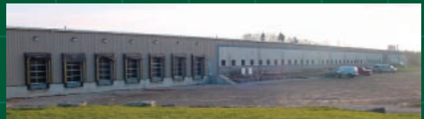
Front view - Plant III
