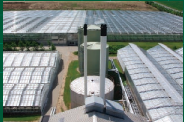
View of Højvang Department and Buffer Tanks
