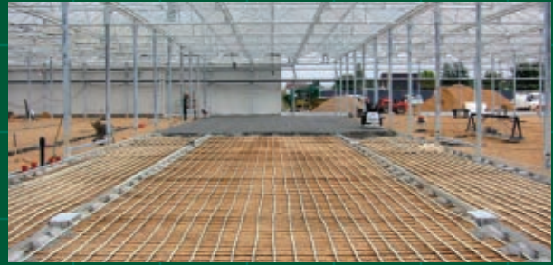
Ebb/Flood Floors Under Construction
